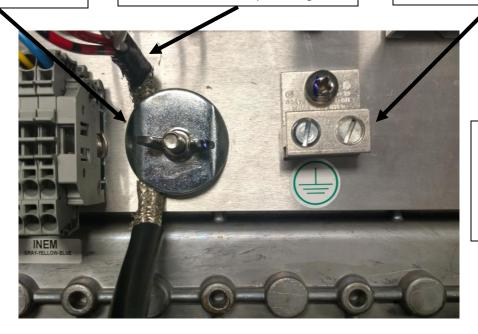
WARNING: Fully tighten wing nut down, DO NOT leave loose. Double check
