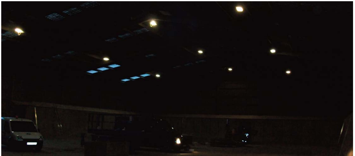
Forth Ports Shed 3 lit by thirteen 400W SON floodlights
