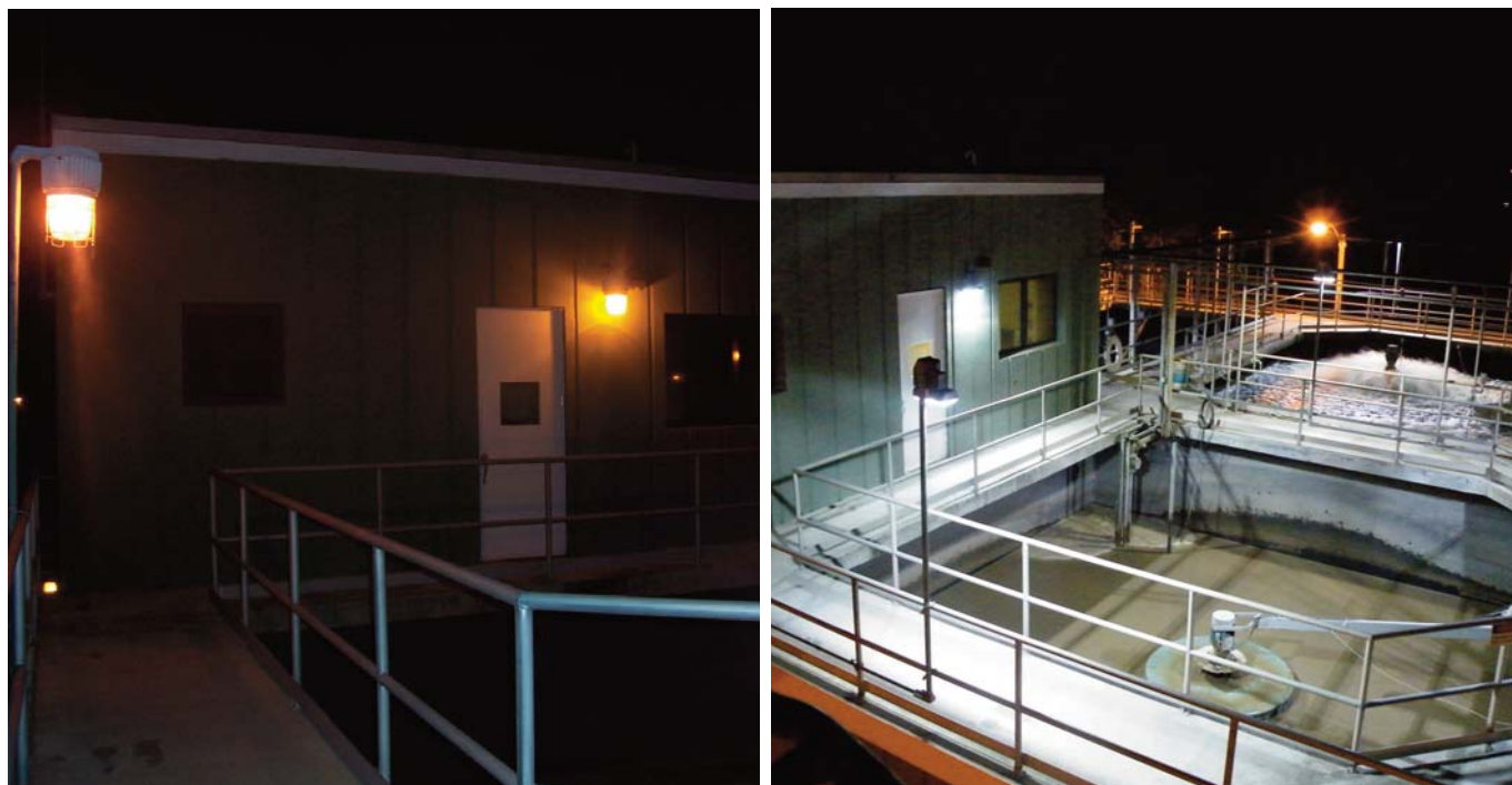
Compare the same scene with HPS lighting on the left and LED lighting on the right.
