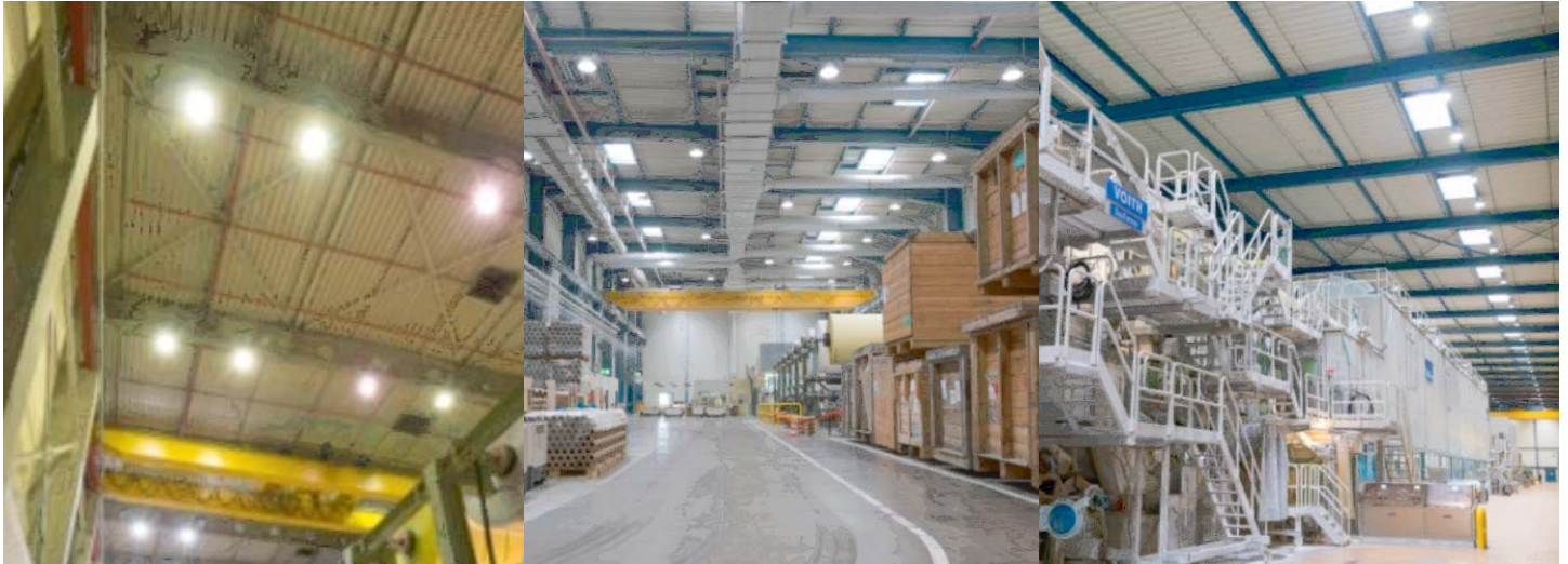
First photo shows 440W metal halide lighting in foreground and LED at back. Two photos on right are lit by 171W LED high bays.
