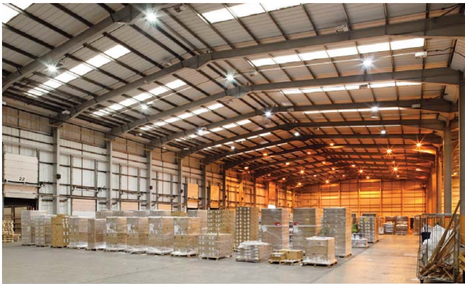
Kuehne + Nagel's Minworth warehouse with 150W Dialight DuroSite LED High Bays in the foreground and 400W HPS fixtures behind.
