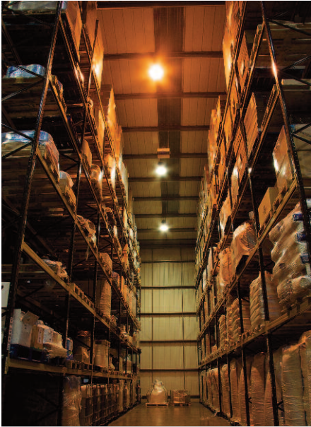
March Foods warehouse lit by HPS on left and then by LED on right.
