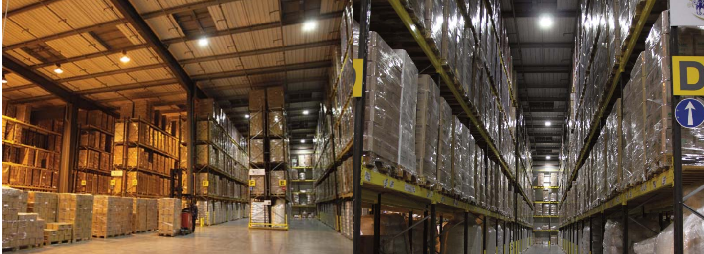
High pressure sodium lighting on the left and Dialight LED high bays on the right.
