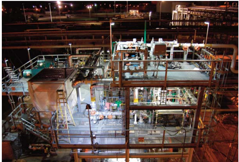
LED lighting installation at the Valero petroleum refinery.
