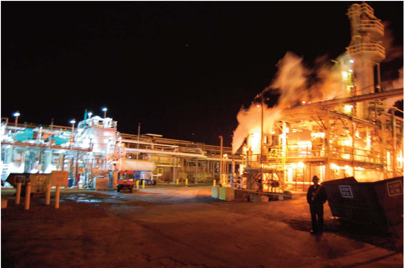
New SafeSite® LED lighting on the left and HPS lighting on the right
