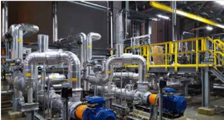
Dialight LED lighting at Rubis Terminal.
