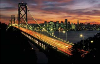
Dialight's LED fixtures can light up bridges where access to change lightbulbs is difficult.
