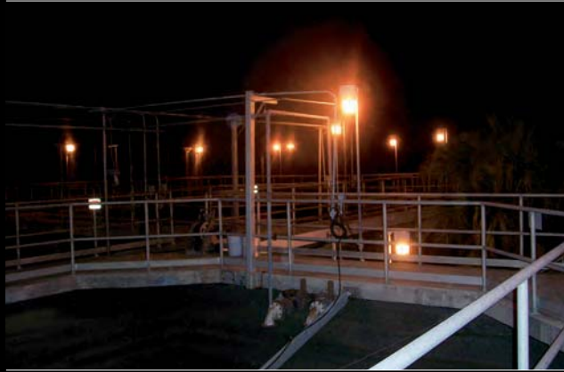
Before Dialight LED lighting was installed
