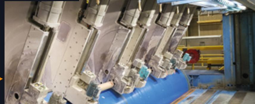
Dialight 4ft low profile linear fixtures mounted under paper machine winders
