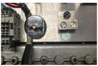
**WARNING:** It is vitally important that the braid and foil be properly connected under the clamping washers for lightning protection. Failure to do will result in premature failures during lightning strikes.
